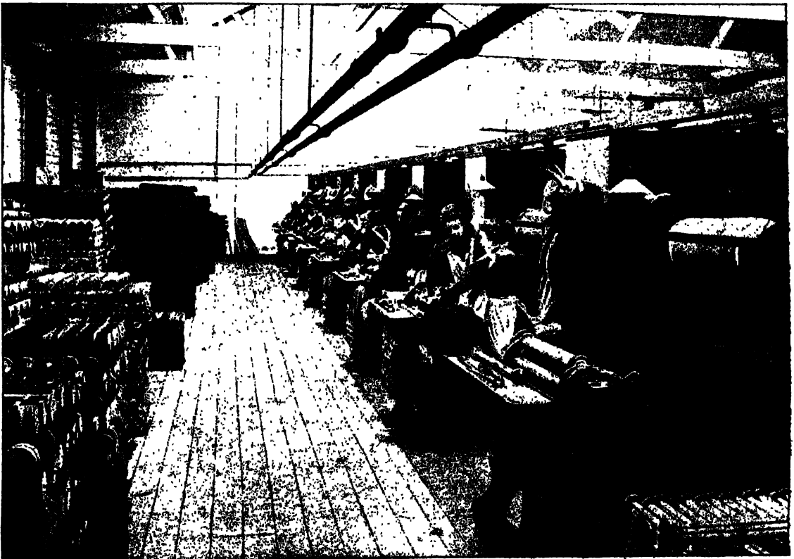
THE "SETTING" DEPARTMENT OF THE CROMPTON AXMINSTER CARPET PLANT (RICHARD SMITH AND SONS).
